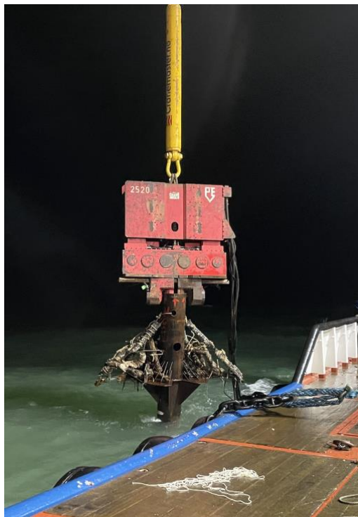
Figure 4: Vibratory hammer used to install eco-anchors offshore in 2022
