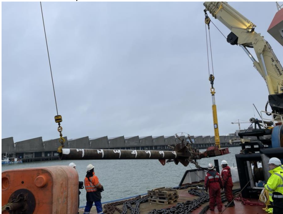
Figure 8: Testing the upending procedure and equipment validation prior to offshore operations
