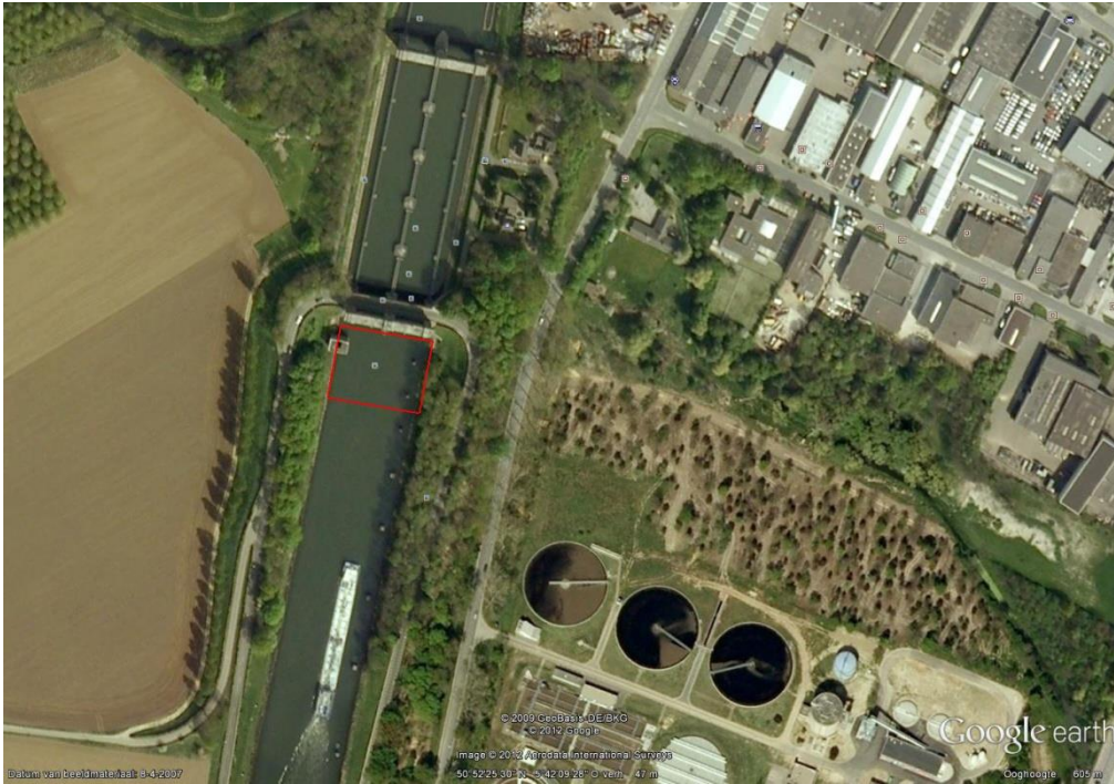
Figure D.7 Areal view of lock Borgharen with the area of the floating debris indicated by a red line.
