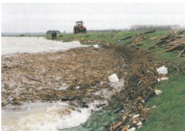
Figure 3.8 Example of floating debris accumulated against a dyke during flood
