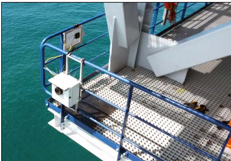
Figure Annex 1-2. Monitoring location Belwind (photo: Belwind).
