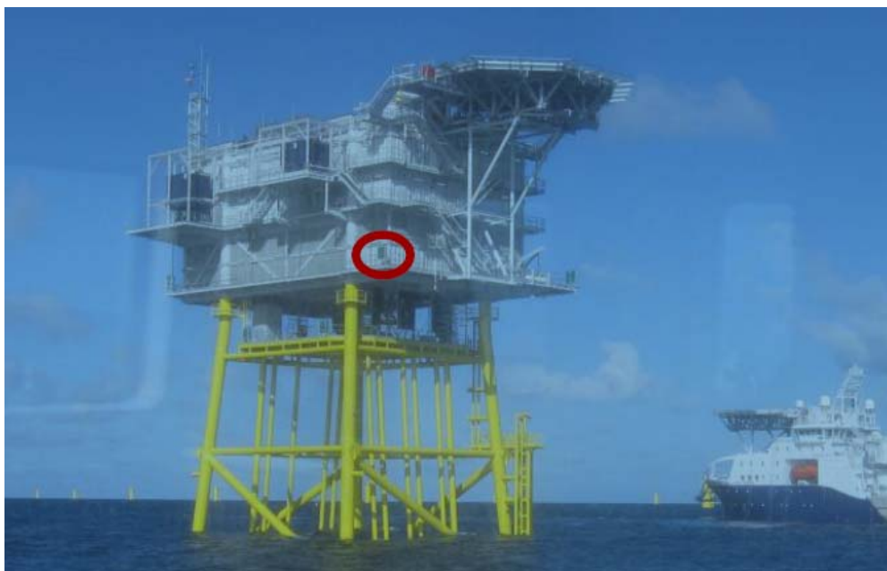
Figure Annex 1-12. Monitoring location Gemini OHVS Buitengaats (photo: Folkert Tazelaar)
